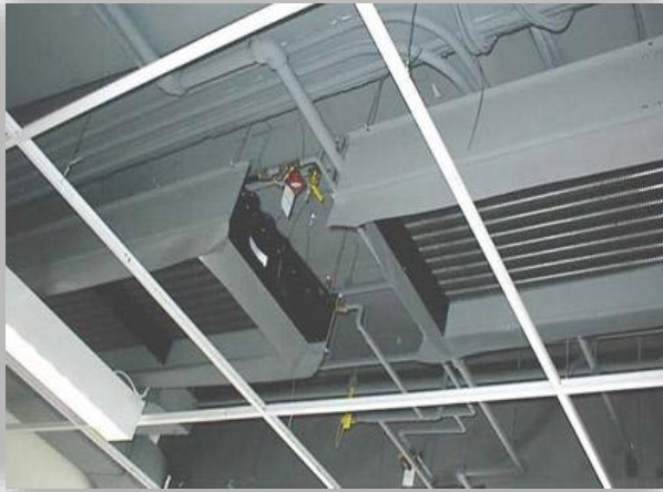
Recessed Passive Beams
